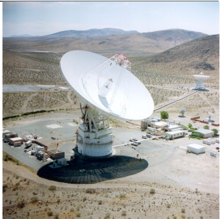
The 70m antenna at Goldstone, California against the background of the Mojave desert. The antenna on the right is a 34m High Efficiency Antenna. The Goldstone Deep Space Communications Complex, located in the Mojave Desert in California, is one of three complexes which comprise NASA's Deep Space Network (DSN). The DSN provides radio communications for all of NASA's interplanetary spacecraft and is also utilized for radio astronomy and radar observations of the solar system and the universe.
