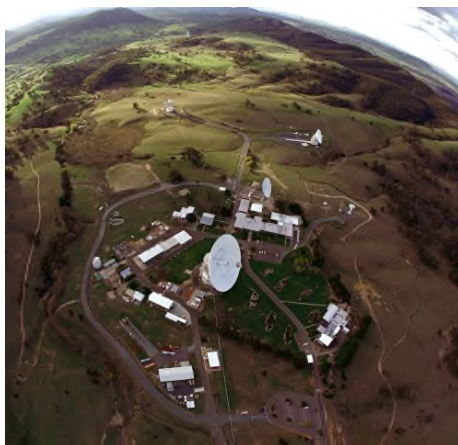
View of the Canberra Complex showing the 70m (230 ft.) antenna and the 34m (110 ft.) antennas. The Canberra Deep Space Communications Complex, located outside Canberra, Australia, is one of the three complexes which comprise NASA's Deep Space Network.
